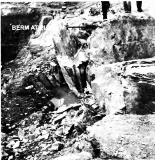
Fig. 3: Effect of toppling in Sandstone at EL 263 m (view to west)
